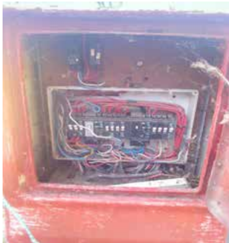
Replacement of the distribution board at the sleeping quarters on the premises of Okkie Jooste cultural facility in Jonkershoek, Stellenbosch.
