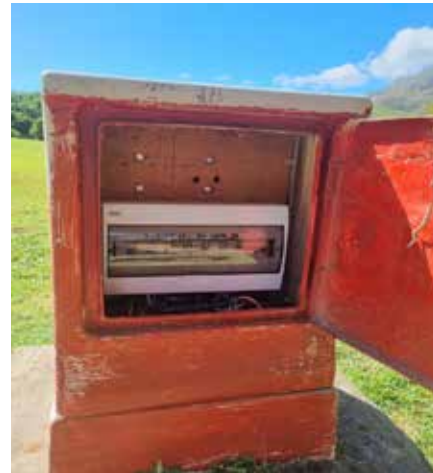
Replacement of the distribution board at the sleeping quarters on the premises of Okkie Jooste cultural facility in Jonkershoek, Stellenbosch.
