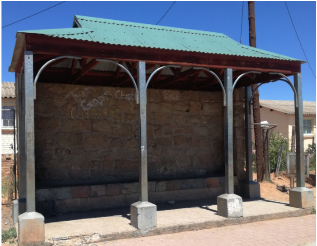
Figure 3-22: Taxi Shelters in Dysselfdorp
